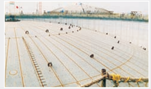
Roof Air Raising
