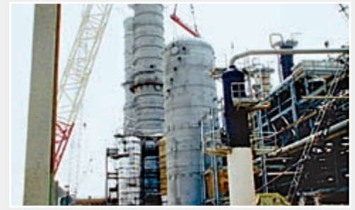
Adsorbent chamber erection
