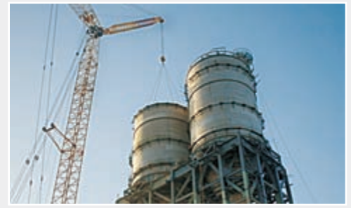
12 metre diameter SS Silo erection on a 45 m elevation platform using a 250 MT Crane.
