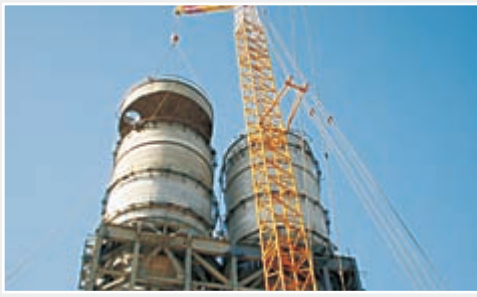
12 metre diameter SS Silo erection on a 45 m elevation platform using a 250 MT Crane.
